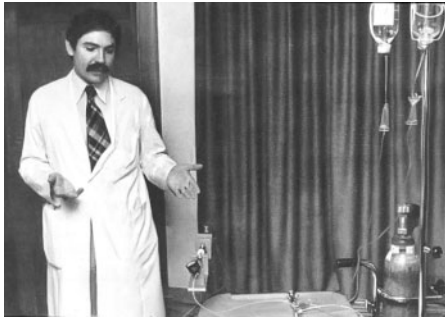
Figure 4 Grüntzig presenting the original pressure inflation device for PCI featuring a pressure gauge and a glass syringe powered by compressed air.
