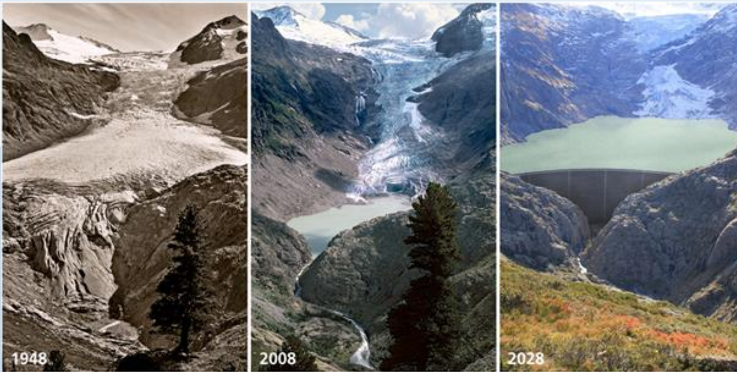
Trift project Oberhasli, CH
