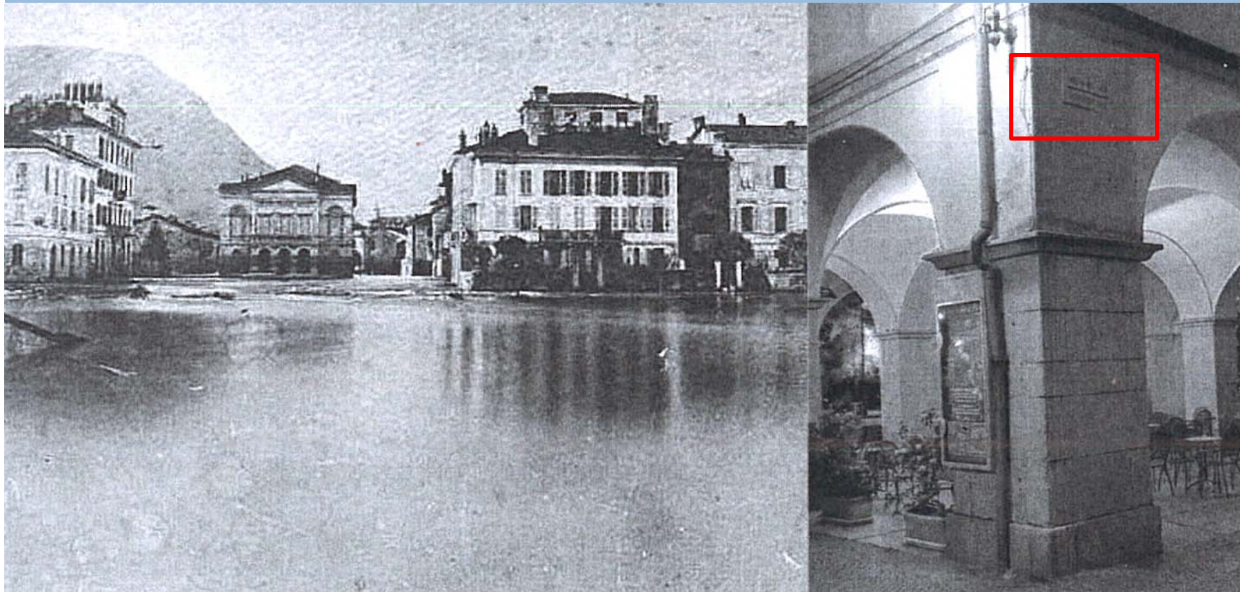
The flood of 1868 in Verbania, Lago Maggiore (left), town arcades with flood mark of 4 Oct. 1868 (right), photographs. Source: Brönnimann et al. 2018: 7.
