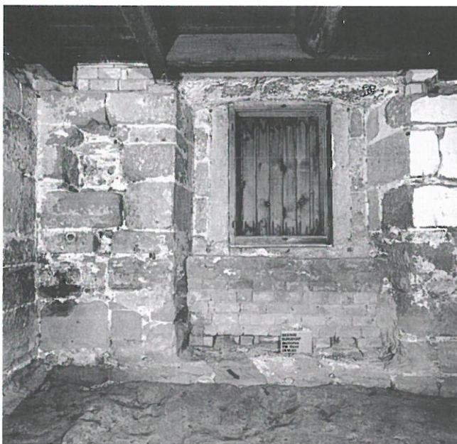
Abb. 19: Conventstube, Fenster in der Westwand.
