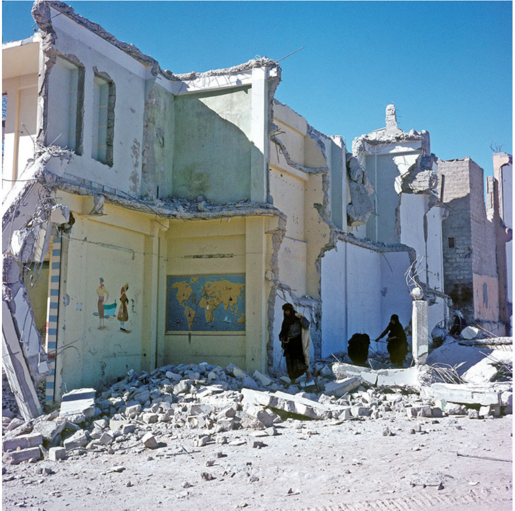
4.15 Tareq S. Rajab, Demolition of New Street , 1962. Color photograph.
