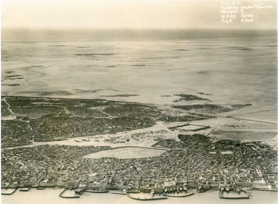
3.1 Aerial view of Kuwait Town. Photograph taken on August 12, 1927.
