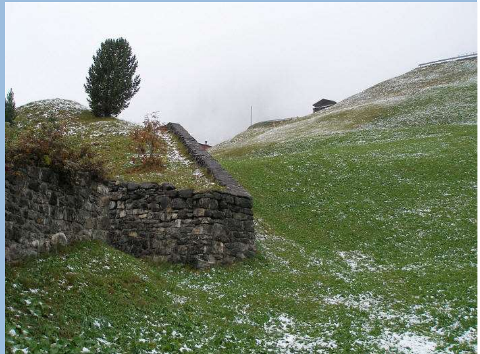
St. Antönien, protective wall against avalanches. Photo by SLF Davos
