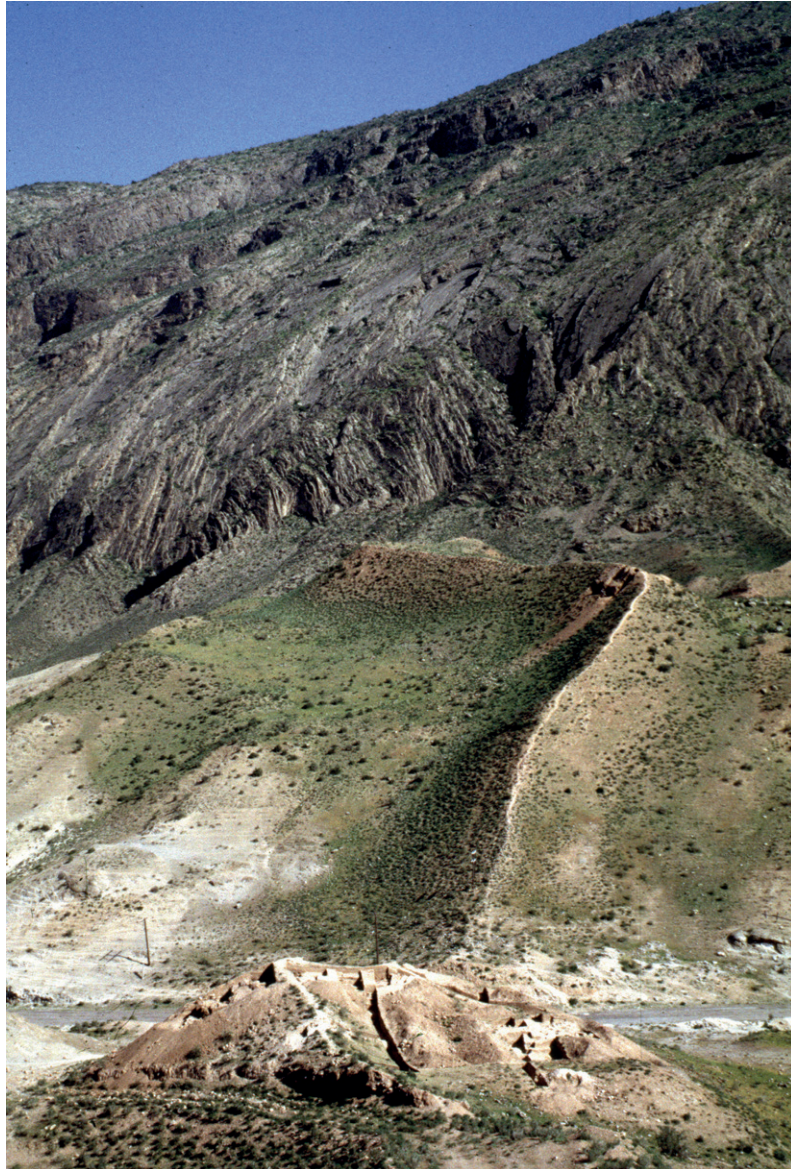
Fig. 16: View of the castle and the wall of the Iron Gates from the south (© MAFOuz-Sogdiane 1997/C. Rapin).
