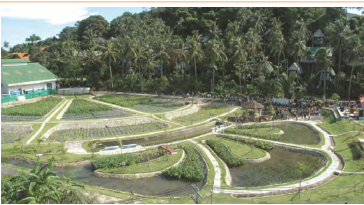
Figure 10: A constructed wetland on Phi Phi Island, Thailand. Without involving stakeholders, such ecological engineering technologies for FSM are rarely adopted or properly used in developing countries. (Photo: Thammarat Koottatep)
