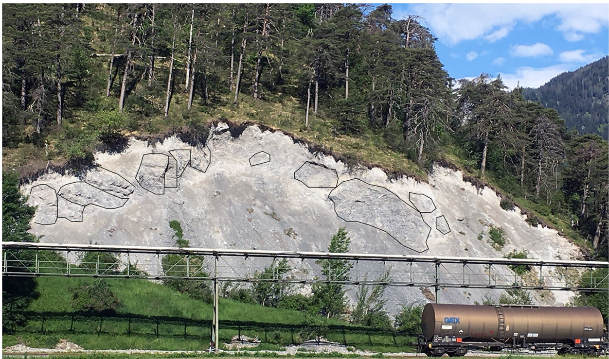
Fig. 7 Outcrop of rock avalanche deposits in the north of Crest'Aulta (coord. 2752.000/1187.800; see Fig. 5B)). Large blocks of limestone at the top of the outcrop rest on finely crushed limestone beneath. Photo A. Pfiffner
