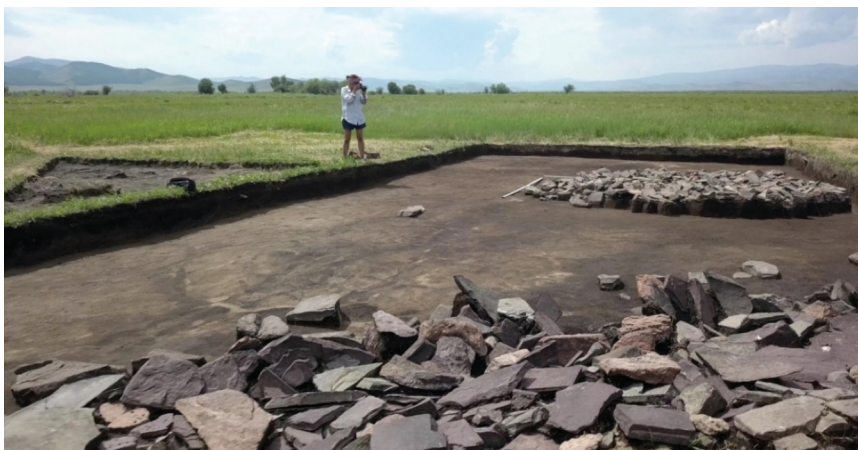
Figure 16. Excavations in the southern periphery of the ‘Tunnug 1’ burial mound revealed funerary structures dating to the 2 nd – 4 th century CE (93°32’50” E, 52°00’25” N) in Tuva Republic, Russia. Photograph credits: Trevor Wallace.
