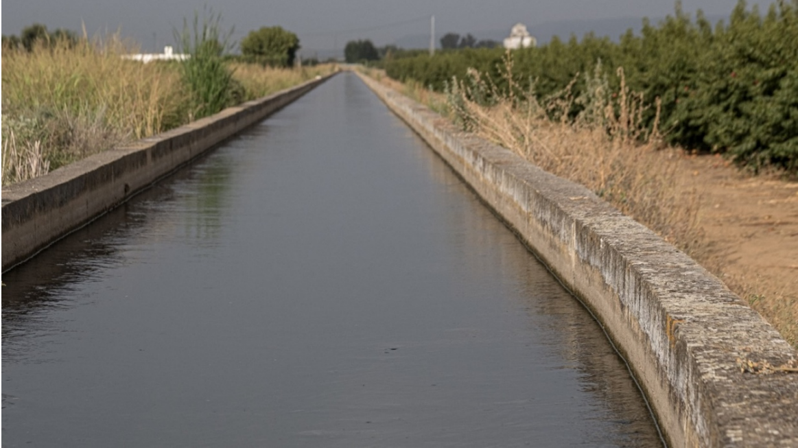
Figure 3. Canal and irrigation system feeding Las Vegas Altas del Guadiana .
