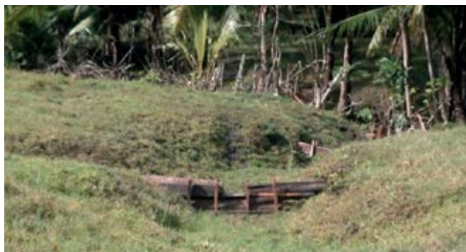
Livestock farm in the province of Los Santos. Gullies plugged with wooden barriers to retain sediments.
