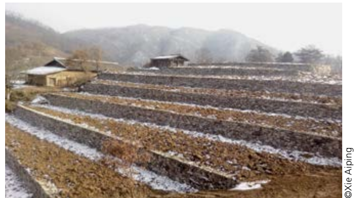
Newly constructed stone dike terraces, Gansu province.
