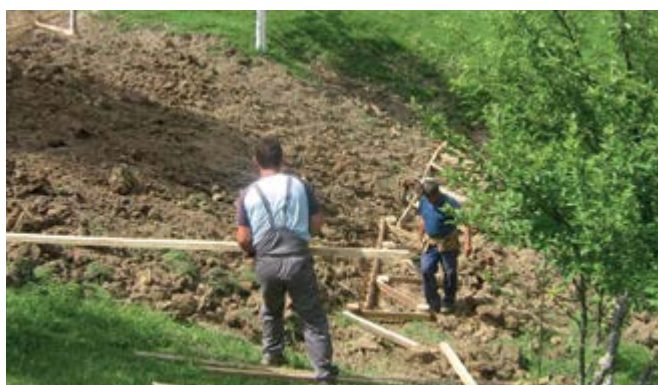
Construction of wooden structures to stop the landslide in Borak, Kladanj municipality.
