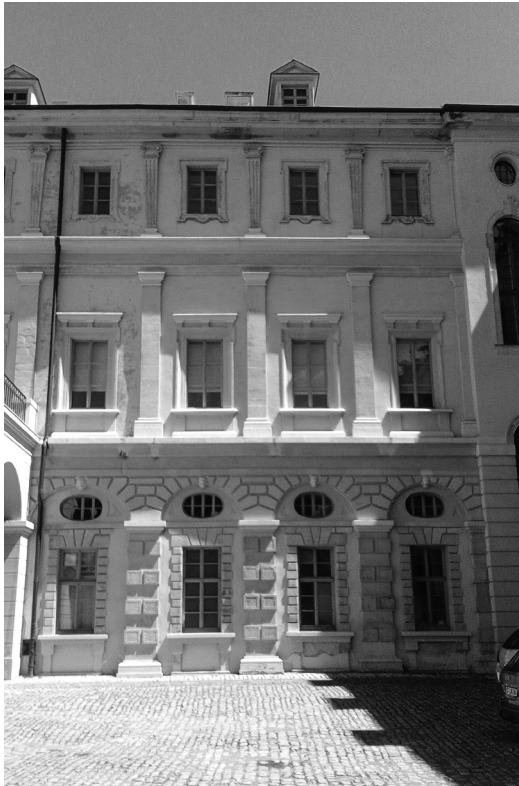
7 Weimar Residenzschloss ; internal façade, south-eastern corner, photographed from the courtyard
