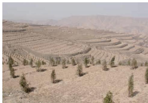
Large-scale application of microcatchments in China. (HP. Liniger)
