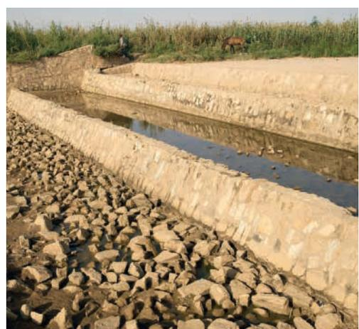
Water spreading weirs built in series (GIZ, 2011).
