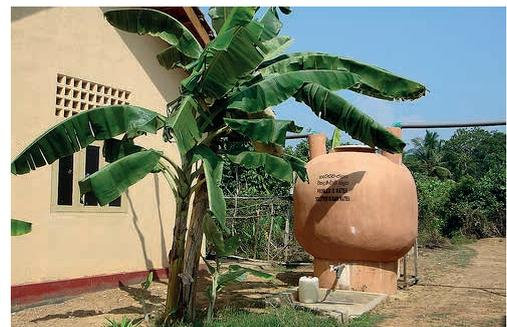
Example of ferro-cement tank, Sri Lanka. (not known)
