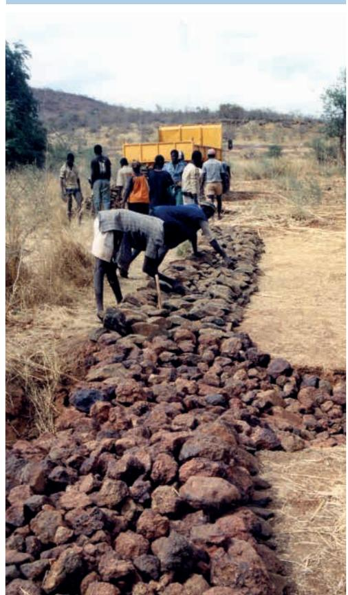
Constructing a permeable rock dam (*digue filtrante*) in Burkina Faso. (W. Critchley)
