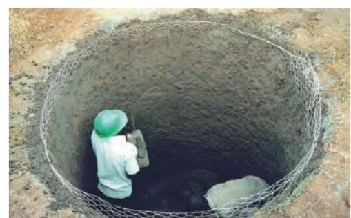
Underground tank for courtyard and road water harvesting, Kenya. This tank was equipped with a silt trap and used for storing runoff (Nissen-Petersen, 2007).
