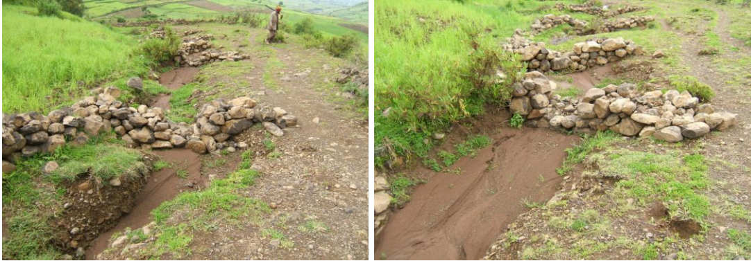
Fig. 30 Series of check dams constructed along path ways
