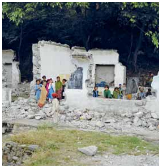
School building demolished by the October 2005 earthquake. Location: Chham, Muzaffarabad District, Azad Jammu Kashmir, Pakistan Photo credit: M.Zimmermann
