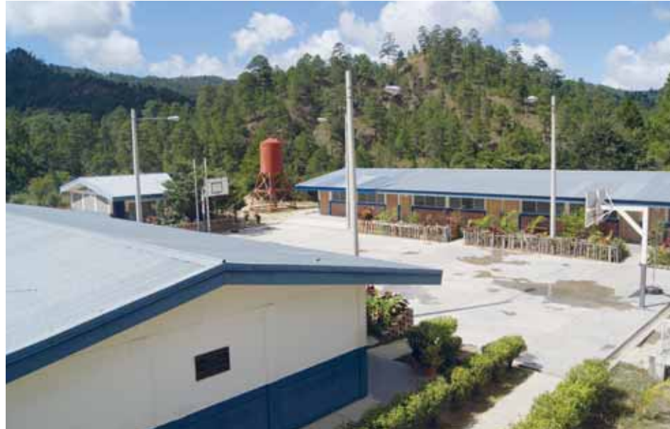
Following risk assessments, it was decided to build the school on safe elevated terrain instead of an initial site potentially exposed to landslides. Location: Dipilto, Nicaragua. Photo credit: SDC Office Managua, Nicaragua
