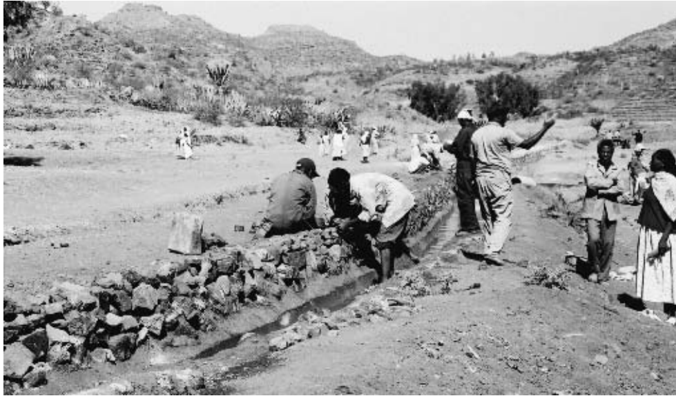
Image 18 Furrow construction for irrigation
