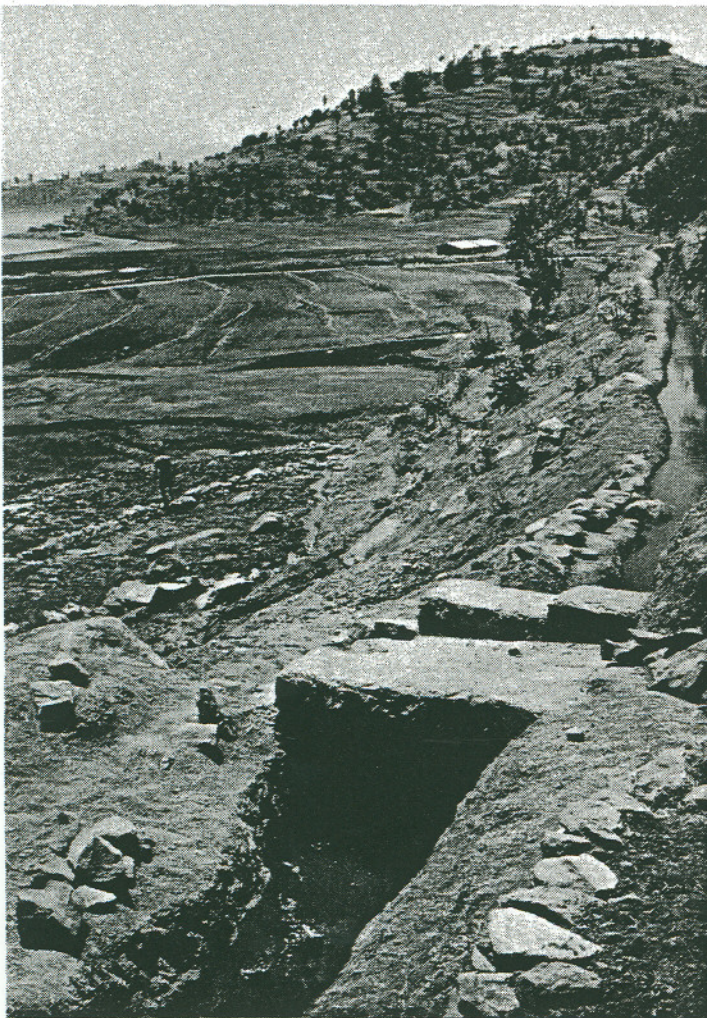
Irrigation structures using natural lakes for periods of insufficient rainfall - a disaster prevention programme as implemented around lake Maybar (Option 2).
