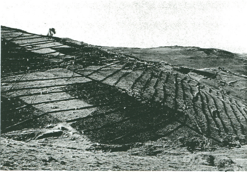
Graded "Fanya juu" conservation measures implemented near Wani Gedel in the Hulet Wenz catchment in December 1983 (Option 2).
