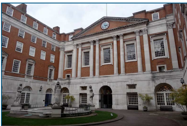
Figure 3. The BMA building.
